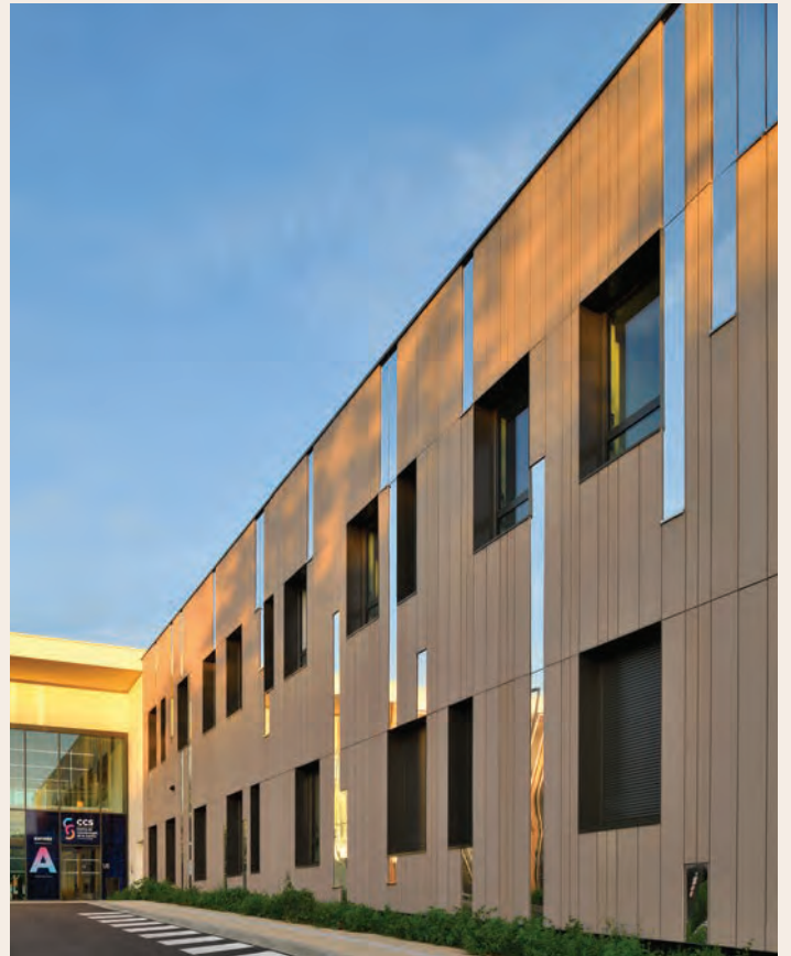
Cancer treatment centre - Le Mans (72) - COVER 14 & 30 - Colour: Sand • Architect: Chabanne • © Photo credit: Erick Sallet
