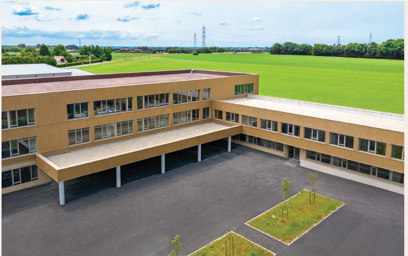
Collège Louise Michel school - Bourneville (27) - COVER 6 - Colour: Sun • Architect: ACAU & AP-MA • © Photo credit: Initial Ingénierie - Matthieu Lecouvey
