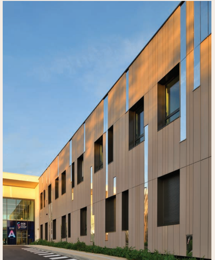
Cancer treatment centre - Le Mans (72) - COVER 14 & 30 - Colour: Sand • Architect: Chabanne • © Photo credit: Erick Salliet
