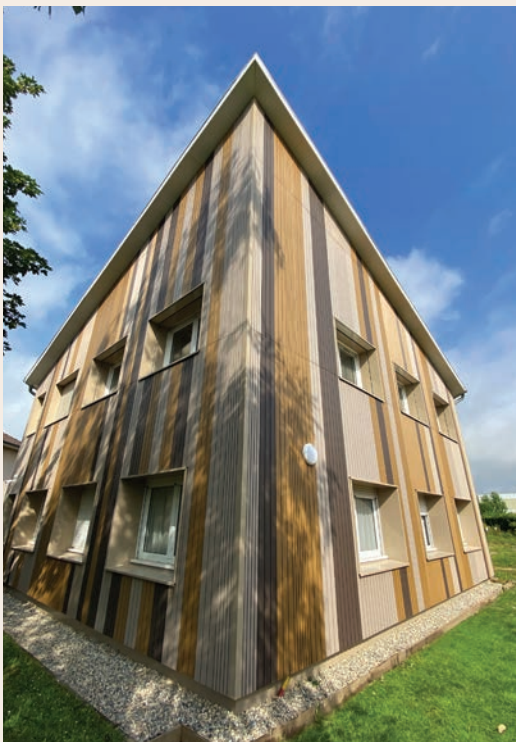
MFR - Moirans (38) - SMART 4 & 9 - Colours: Sun, Sand & Earth • Architect : Dedale
