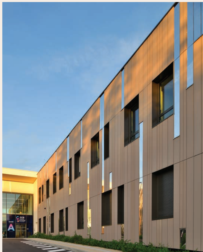
Cancer treatment centre - Le Mans (72) - COVER 14 & 30 - Colour: Sand • Architect: Chabanne • © Photo credit: Erick Salliet
