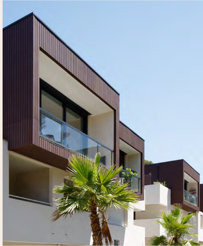
Multi-unit housing - Quinta Coliba - Marseilles (13) - SMART 9 - Shade - Heat Architect: MAP Architecture
