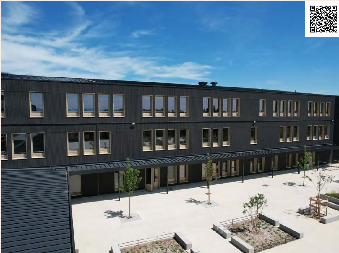
Collège Simone Veil - Saint Priest (69) - COVER 6 - Shade - Night • Architects: Aurélie Dargnat / Sarah Bigot for the City of Lyon
