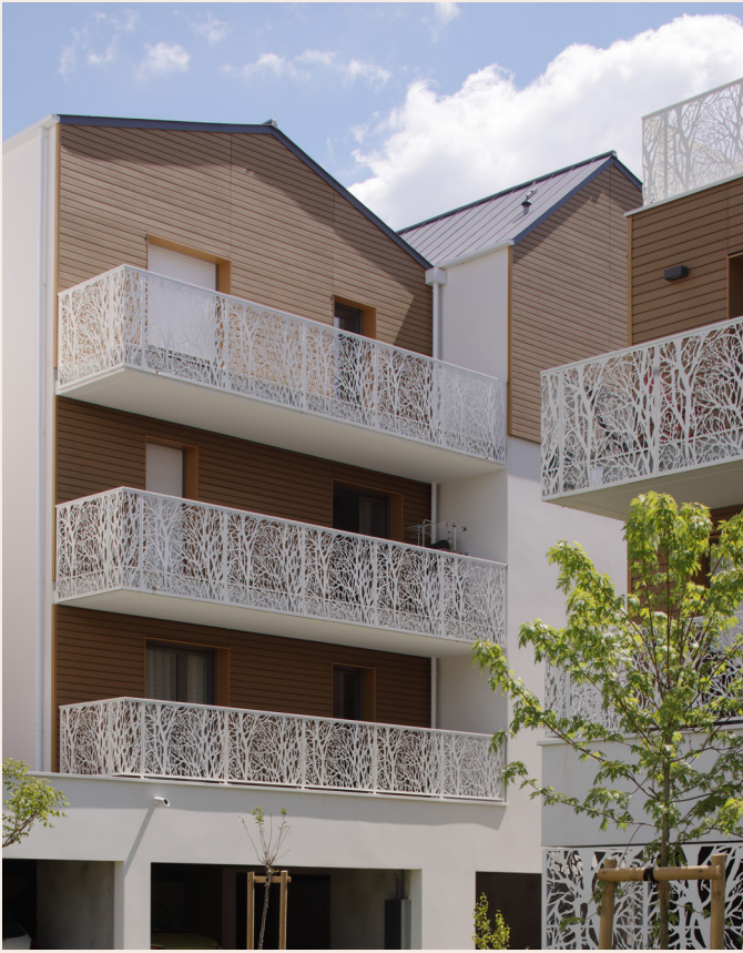
Multi-unit housing - Le Carré Silva - St Herblain (44) - SMART 9 - Shade - Sun Architect: Mark Guegan / Atelier 2G
